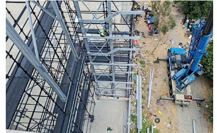
Curro Foreshore, Kaapstad
